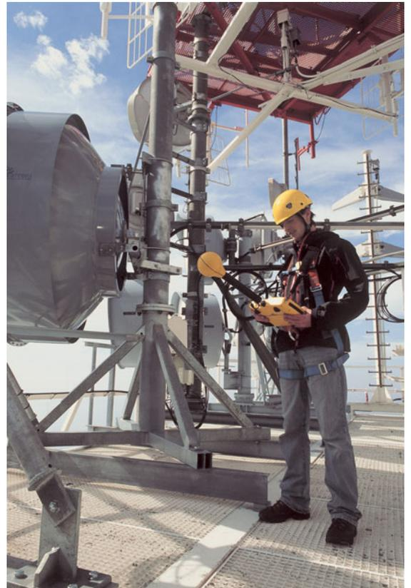
**Figure 6: The often large numbers of antennas installed on radio masts mean that measurements must be made to check safety on the various platforms.**
